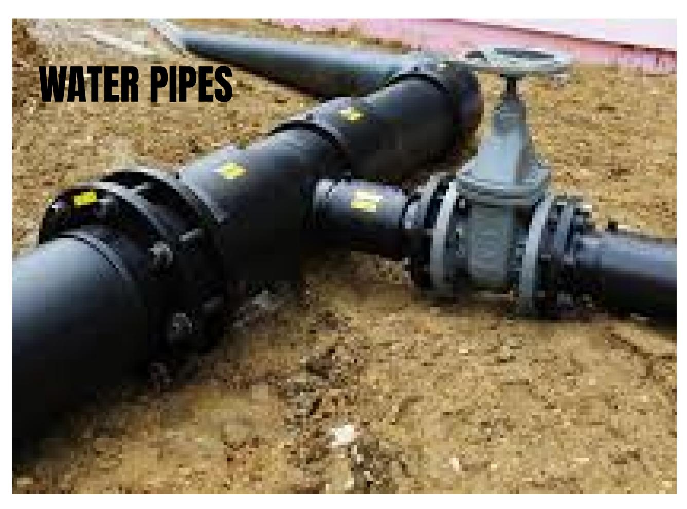
HDPE PE100 pipe is easy to install, light, flexible, corrosion-free and has a service life of up to 50 years. It can be jointed using butt fusion or electro-fusion to create a leak-free pressure network for water. Major application areas are: Metropolitan Water Supply System, Civil Engineering, Construction, Building, Agriculture, Industrial, Mining, Marine/Aquaculture and Water & Oil Boring.
